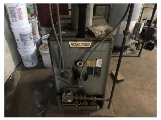
Natural gas-fired boiler in sub-basement used to heat adjoining sidewalks (ice & snow removal). Eight 5-gallon buckets of anti-freeze used in the sidewalk deicing system.
