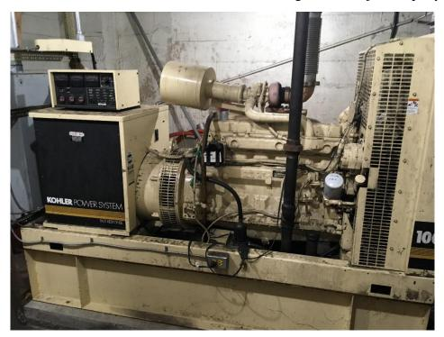
Emergency back-up electrical generator, with integral diesel fuel AST located in the sub-basement.
