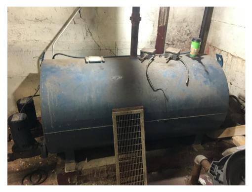
Aboveground storage tank (AST) of makeup water for the natural gas-fired steam boiler located in the sub-basement and used to heat the main building on the Subject Property.
