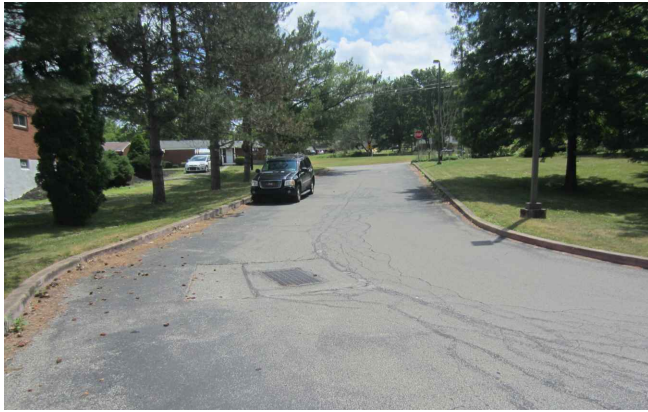
PHOTO 1 AREA TO BE CLEANED, SEAL CRACKS, AND SEAL AREA. RE-ESTABLISH FLOW LINE FOR DRAINAGE
