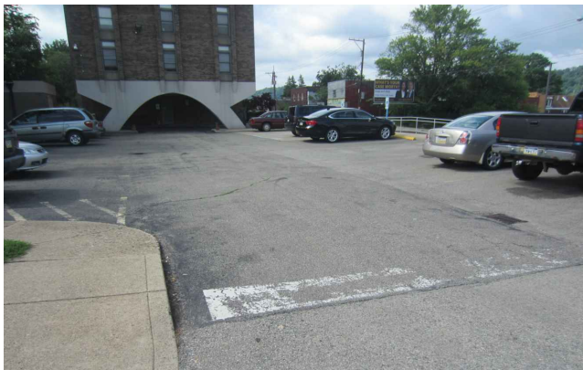
PHOTO 3 PARKING AREA TO BE RELINE STRIPED, CLEANED AND SEAL CRACKS, AND SEAL ASPHALT
