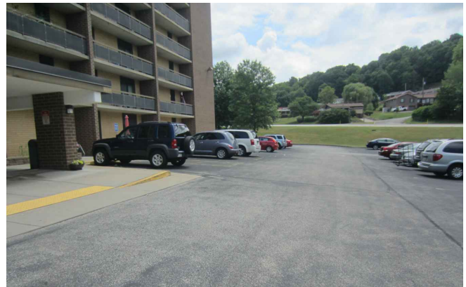
PHOTO 6 PARKING AREA TO BE CLEANED, SEAL CRACKS, AND SEAL PARKING AREA
