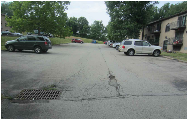
PHOTO 3 800 SF TO BE MILLED AND RESURFACED
