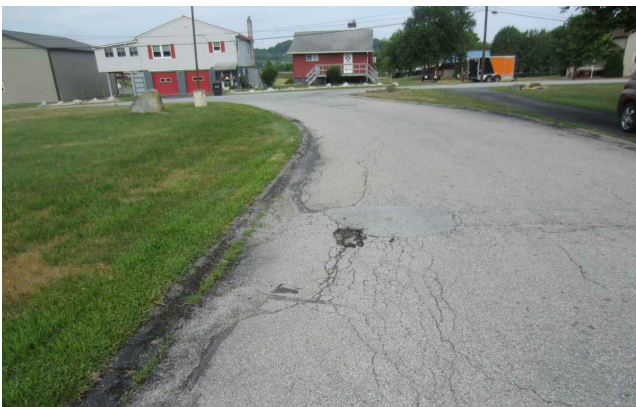
PHOTO 3 100 SF TO BE MILLED AND RESURFACED
