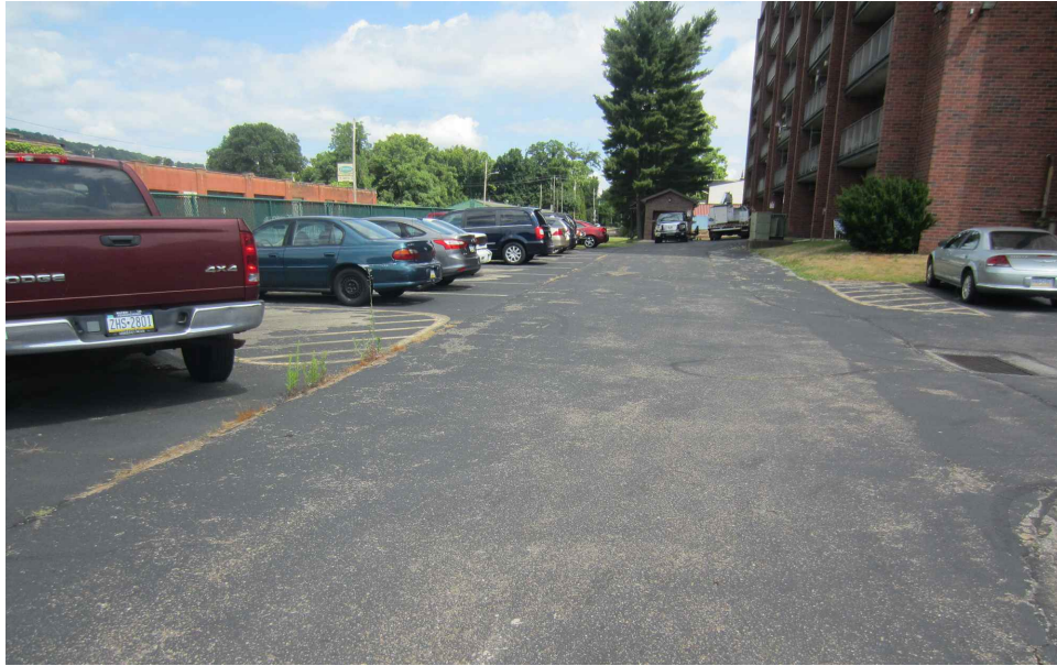
PHOTO 1 34 PARKING SPACES TO BE RELINED STRIPED, CLEAN AND SEAL CRACKS, AND RESEAL ASPHALT
