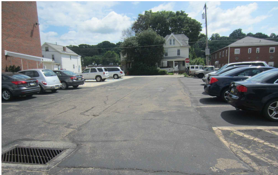
PHOTO 2 34 PARKING SPACES AND 4 HANDICAP PARKING SPACES TO BE RELINE STRIPED, CLEAN AND SEAL CRACKS, AND RESEAL ASPHALT
