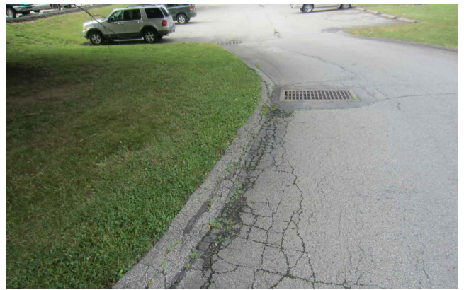
PHOTO 2 20 LF OF CURB TO BE MILLED AND RESURFACED
