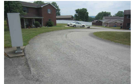
PHOTO 6 2,700 SF TO BE MILLED AND RESURFACED
