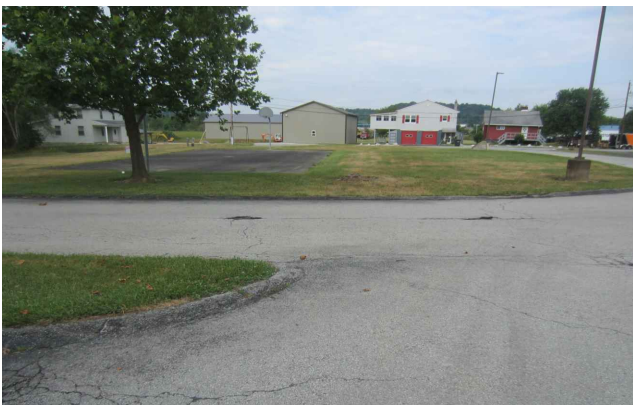
PHOTO 5 120 SF TO BE MILLED AND RESURFACED
