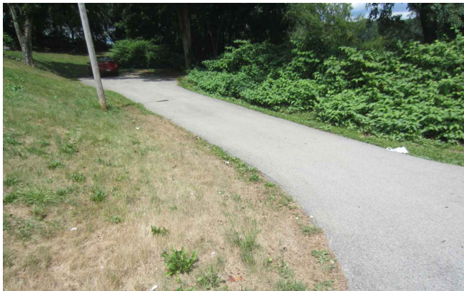
PHOTO 3 PARKING AREA TO BE CLEANED, SEAL CRACKS, AND SEAL PARKING AREA
