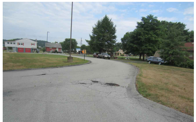
PHOTO 6 120 SF TO BE MILLED AND RESURFACED
