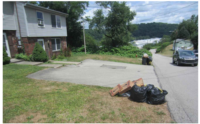
PHOTO 2 PARKING AREA TO BE CLEANED, SEAL CRACKS, AND SEAL PARKING AREA
