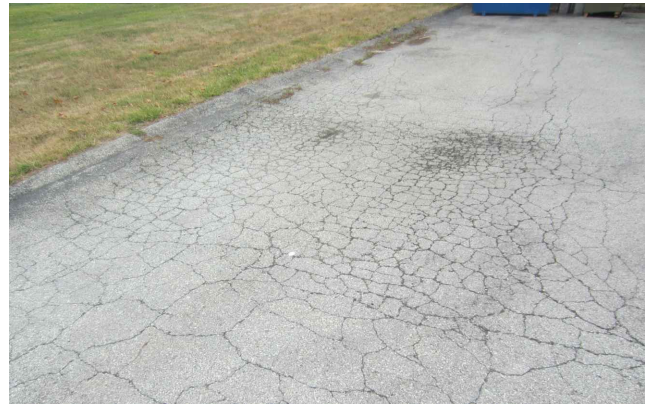
PHOTO 8 200 SF TO BE MILLED AND RESURFACED
