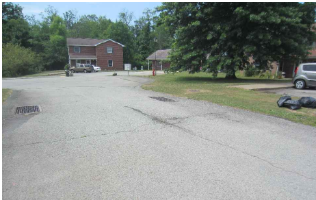
PHOTO 5 160 SF TO BE MILLED AND RESURFACED
