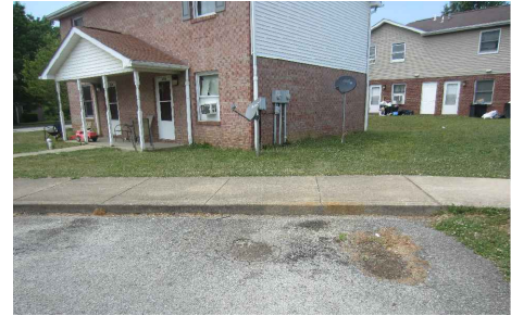
PHOTO 4 160 SF TO BE MILLED AND RESURFACED
