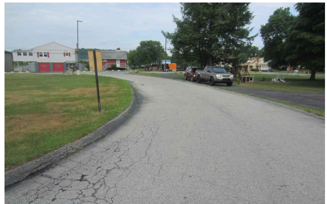
PHOTO 4 60 SF TO BE MILLED AND RESURFACED
