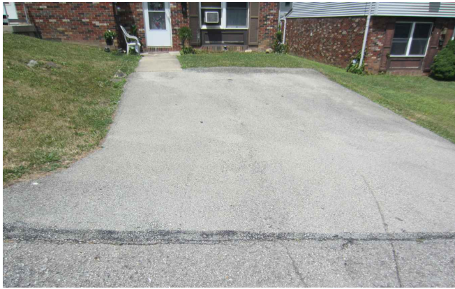
PHOTO 1 PARKING AREA TO BE CLEANED, SEAL CRACKS, AND SEAL PARKING AREA
