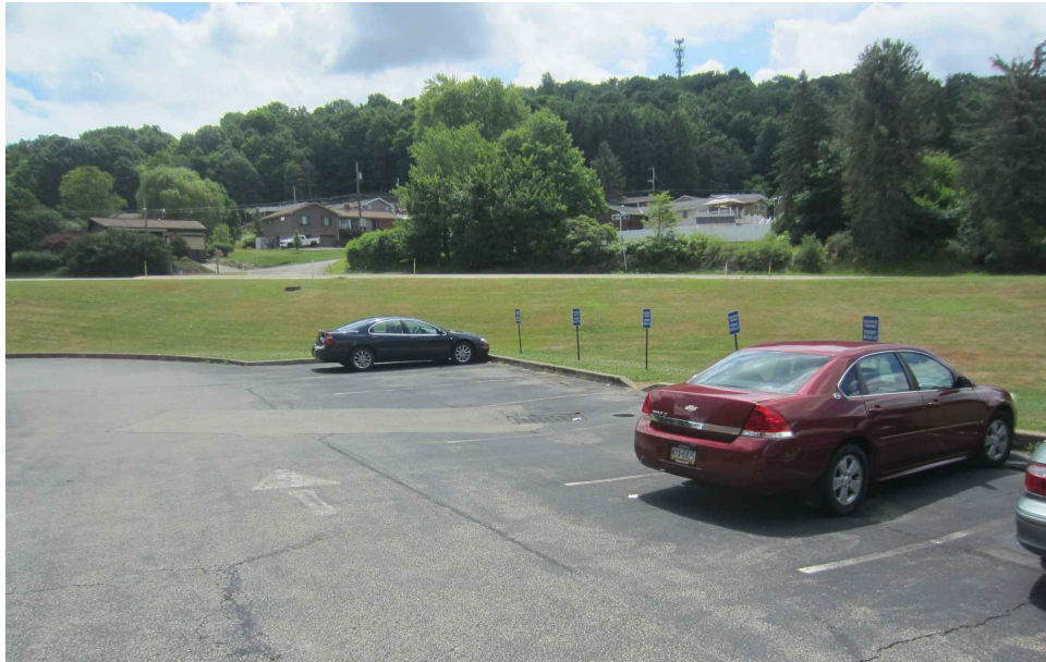
PHOTO 7 PARKING AREA TO BE CLEANED, SEAL CRACKS, AND SEAL PARKING AREA
