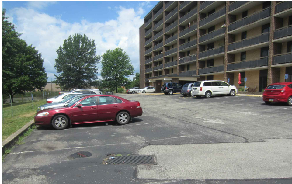
PHOTO 8 120 SF SOFT SPOT TO BE REPAIRED. RE-ESTABLISH FLOW LINE TO INLET. PARKING AREA TO BE CLEANED, SEAL CRACKS, AND SEAL PARKING AREA
