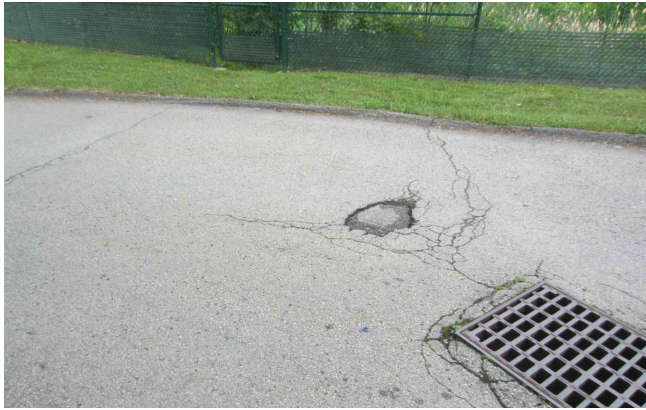
PHOTO 1 25 SF TO BE MILLED AND RESURFACED
