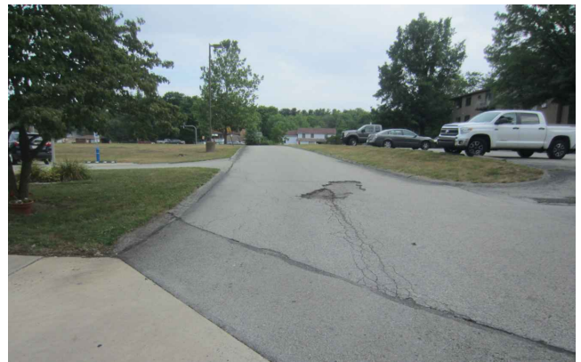
PHOTO 10 96 SF SOFT POT AREA TO BE REPAIRED
