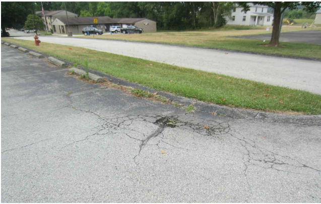
PHOTO 7 16 SF TO BE MILLED AND RESURFACED
