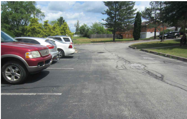
PHOTO 3 120 SF SOFT SPOT REPAIR AROUND INLET. PARKING AREA TO BE CLEANED, SEAL CRACKS, AND SEAL PARKING AREA. RE-ESTABLISH FLOW LINE FOR DRAINAGE
