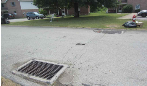
PHOTO 3 250 SF TO BE MILLED AND RESURFACED FROM THE MIDDLE OF THE ROAD AND AROUND THE INLETS
