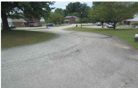
PHOTO 7 2,700 SF TO BE MILLED AND RESURFACED
