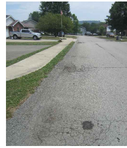
PHOTO 2 8'X20', 160 SF TO BE MILLED AND RESURFACED
