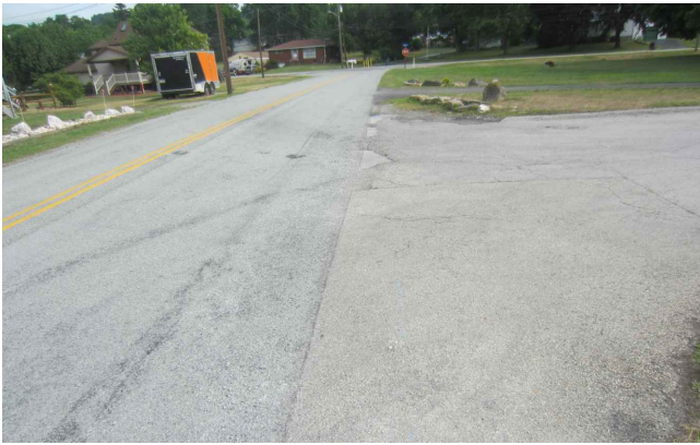
PHOTO 1 304 SF TO BE MILLED AND RESURFACED
